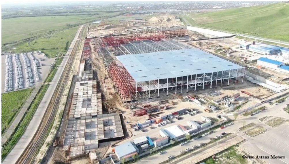
Figure 8 – Photo of the construction of the Astana Motors Manufacturing multi-brand plant in Kazakhstan Notice – compiled by author based on the source [1]
